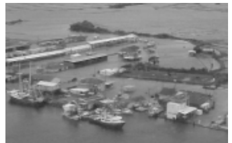
Following Tropical Storm Isidore, the natural boundary between land and water along LA 1 in Leeville was seemingly nonexistent.
