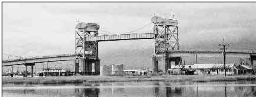
Existing Lift-Bridge over Bayou Lafourche at Leeville
